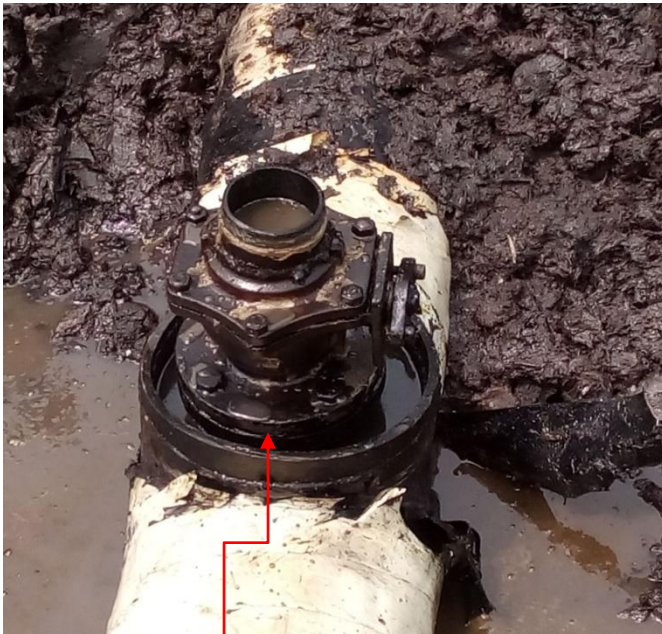
Fig B: Incident Facility
