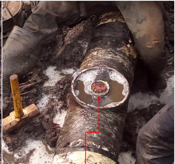
Fig C: Incident Facility during repair
