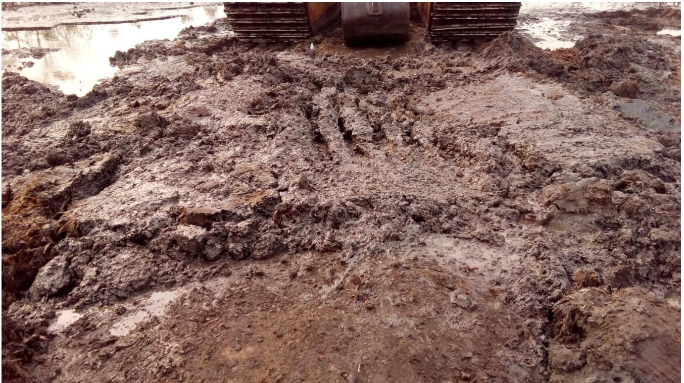
Fig F: Backfill after repair of incident facility
