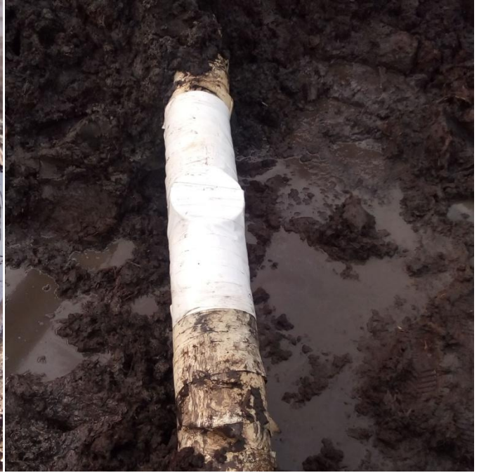
Fig E: The Spill Point after repair
