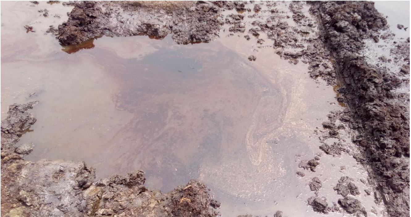
Fig A: The Leak point just before excavation
